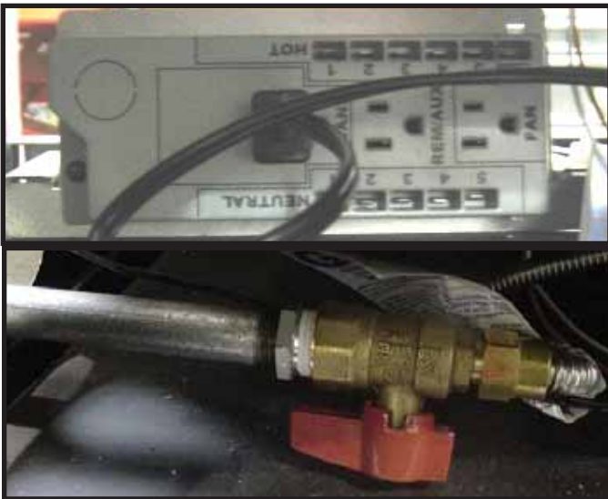
Figure 13.1 Preparation to Install Splatter Guard
